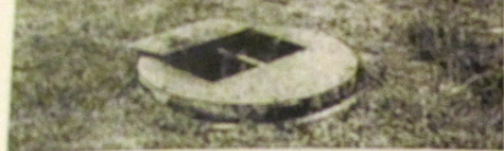
Lafollette #2 looking towards Kings Hill Lift Station
